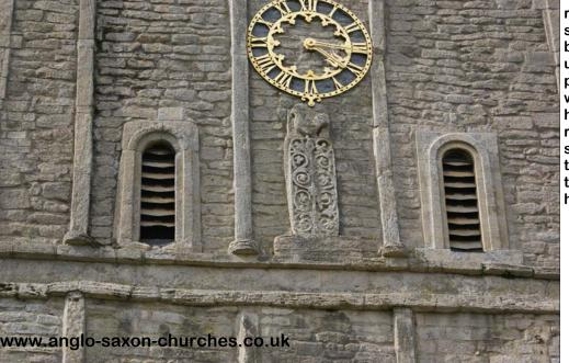
random quoin stones but the second stage has long-and-short work and is cut back to allow a plaster covering to be run up against the upstanding edge (see picture). This should be bore in mind when viewing the windows which would have shown as the upstanding 'rib' around the window running and surrounded by plaster rendering covering the main surface of the walling. It seems there are two stages/dates of building here.
